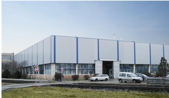
Caption picture 1: Concrete sleeper factory of TRAVERTEC S.R.L. in Buzau (Romania) (Photo: PCM RAIL.ONE AG).
